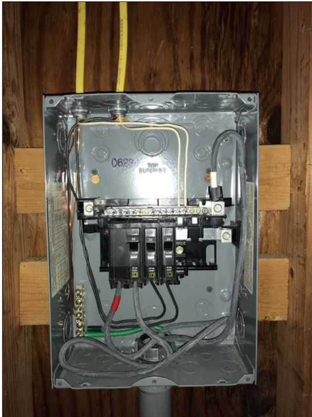
Panel and detached shed
