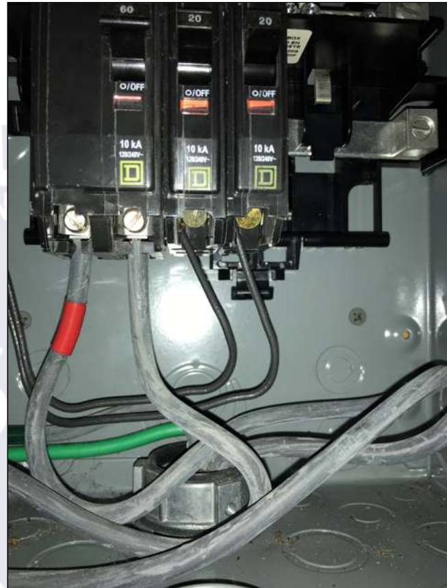
Panel and detached shed
